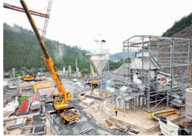
Plant under construction
