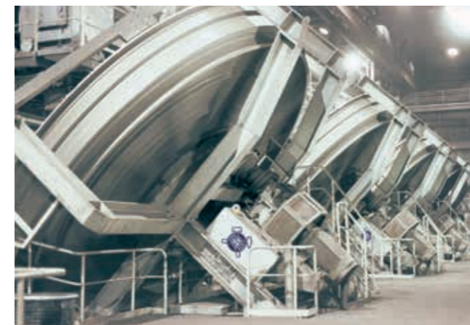
Pelletizing plant, iron ore, 140t/h, HAVER SCARABAEUS
